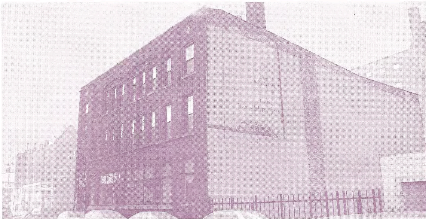
Three Walls - 119 N Peoria St.
